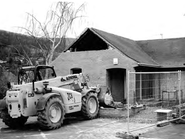
Mayfair in February – the builders arrive
