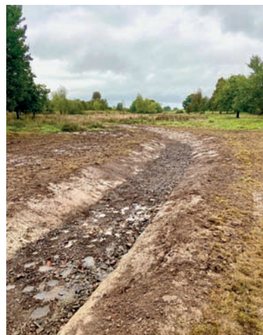
The new riverbed being constructed in Coppice Leasowes
